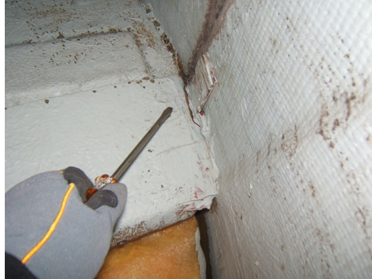
Main beam starboard side
